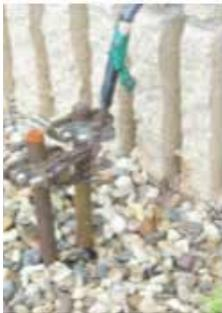
A system ground is ground rod(s) bonded together and connected to the power supply of the system. Ground rods can be metallic spikes driven into the ground, rebar, structural building
