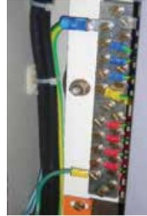
require additional equipment grounds for proper operation. These grounds must be connected at a single point to the ground. Electronic equipment cannot have separate system grounds.
