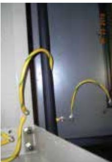
Equipment grounds must provide a path from the equipment to the system ground. Equipment grounds can be conductors, metallic conduit, or cable raceways.
