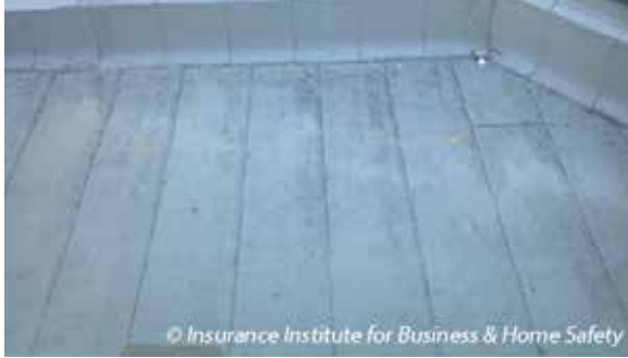
Modified bitumen roof cover.
