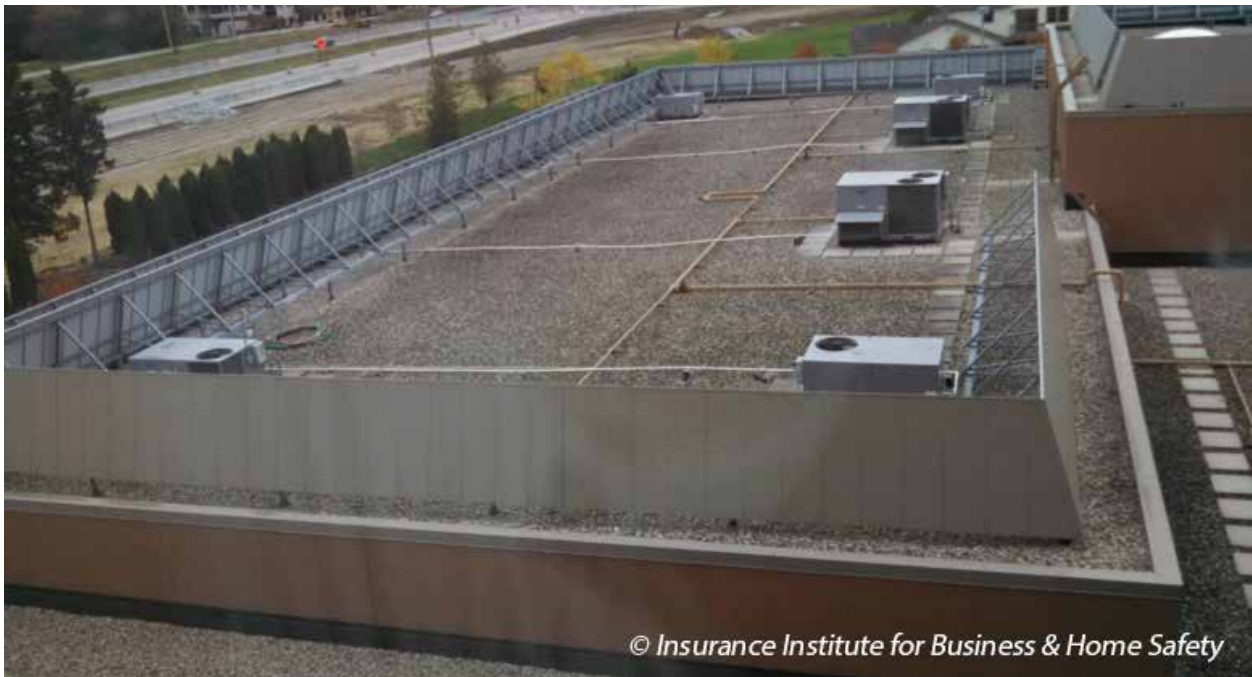
A wind screen on a low-sloped ballasted roof concealing rooftop equipment from the street and neighboring buildings.
